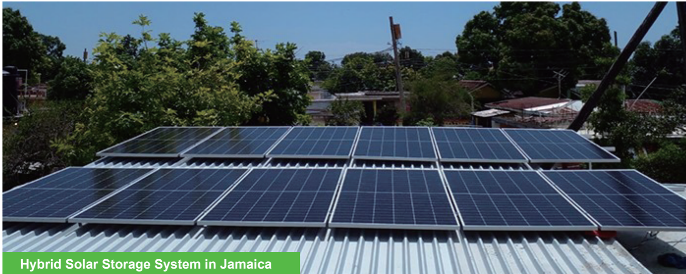
Jamaica household solar storage project
